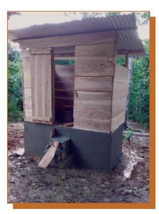
cement- block base built off the ground. Inside, are two adjacent holes where a cement-molded seat stands over one of them. The system separates the urine from the dry matter, converting excrement into fertilizer after about 4 months. It serves a dual purpose.
